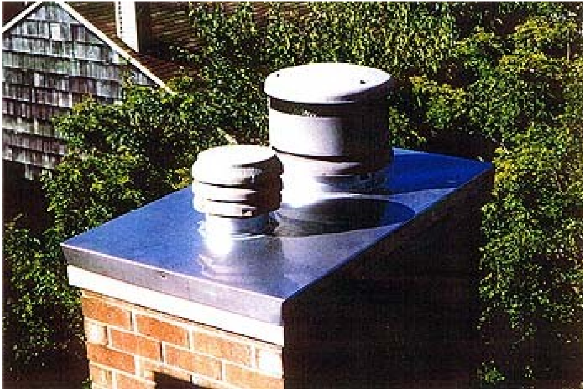
Picture after new chase cover installed
