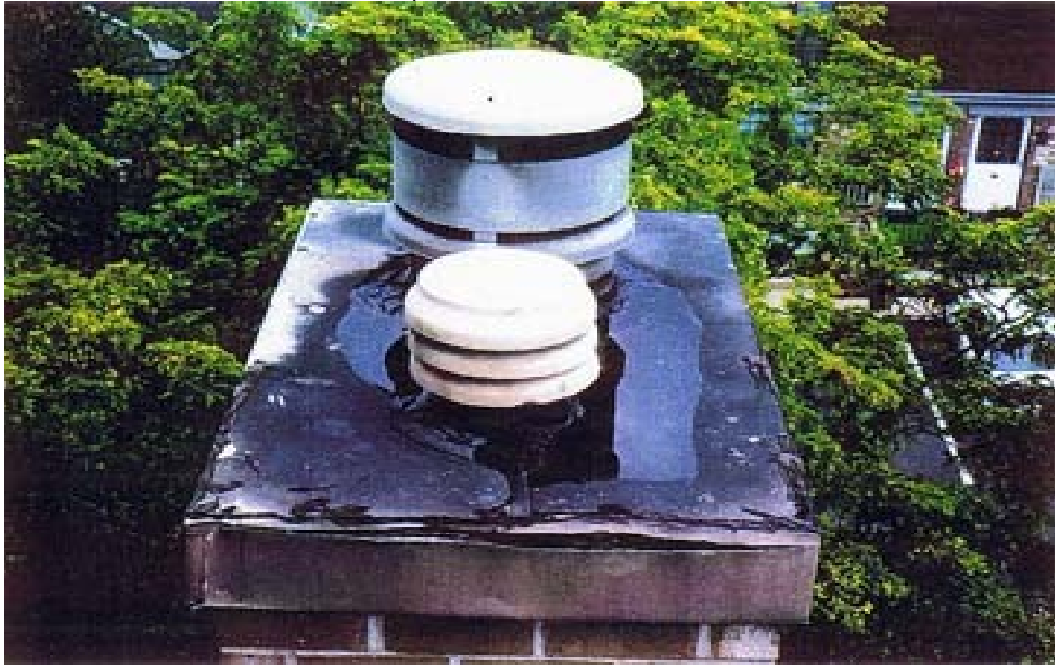
Picture after new chase cover installed
